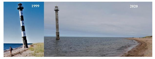
**Figure S1.** Location of Kiipsaare lighthouse (height 25 m) in relation to the shoreline in 1999 and 2020 (photos: Ü. Suursaar).
